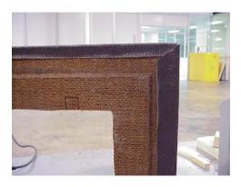
11. Wrapping the panel is continued along all three edges of the panel. To complete the wrapping of this entire dado panel took approximately 15 minutes. All hardware can then be reattached to the dado panel to produce a finished part.
