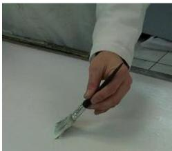
4. It is important to apply the contact adhesive uniformly and evenly since "heavy" application areas will take longer to dry and may cause delamination if material is applied while parts of adhesive are still wet. Allow the adhesive to dry so that it becomes tack-free per the manufacturer's instructions. If using a water-based adhesive, drying time will be longer than using a solvent-based adhesive.
